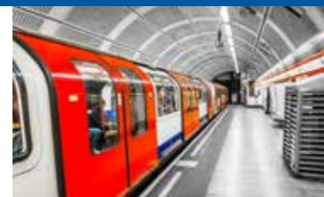
...in underground railways
